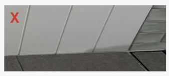
Panel used in a bathroom not installed on top of a skirting resulting in water wicking up the bottom of the panel and damaging it  $\frac{1}{2} \int_{-\infty}^{\infty} \frac{1}{2} \left( \frac{1}{2} \int_{-\infty}^{\infty} \frac{1}{$
