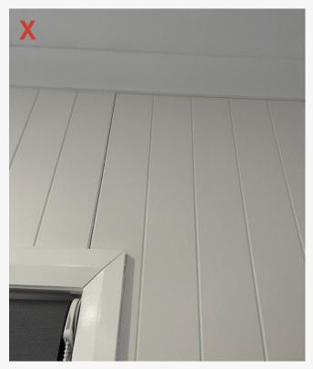
Tongue and groove join showing due to no flexible paintable sealant being used  $\label{eq:constraint} % \begin{center} \begin$
